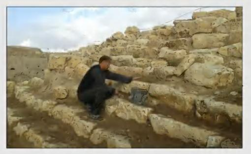
we must then each spring re-fill the joints between the stones with mud: this keeps the stones from becoming loose and the staircase from falling apart
